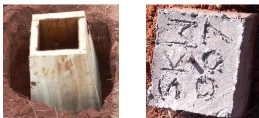
Plate 3.2: Model of Short Truncated Pillar and Monumented new control pillar (SKW 007) at Vuga market.
